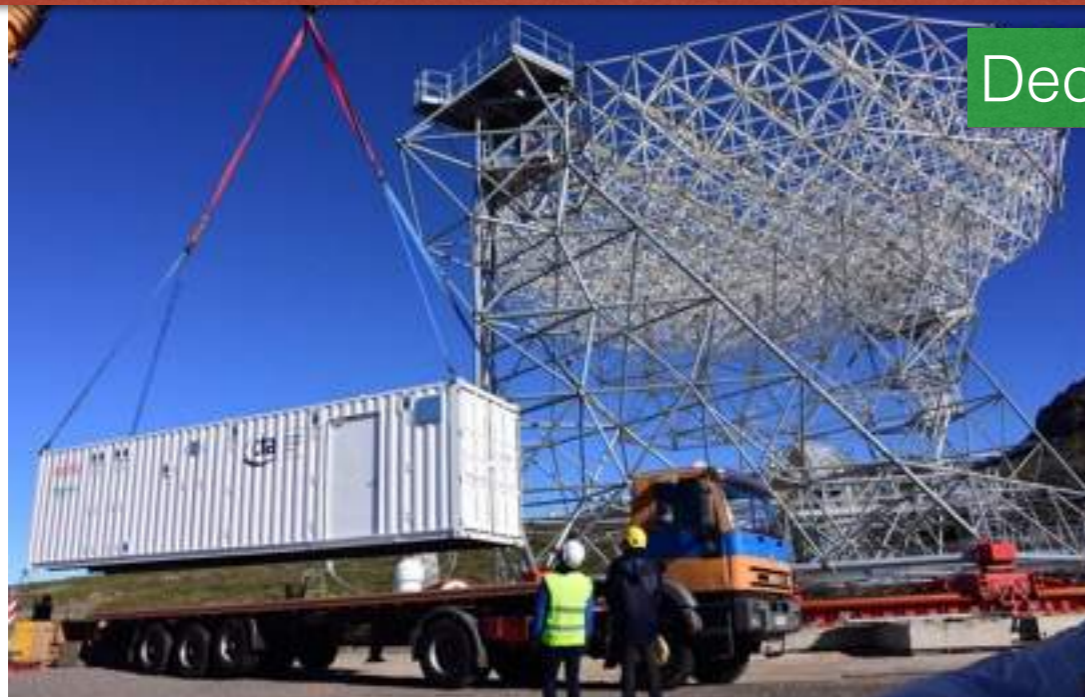
Onsite IT computer center physically installed
